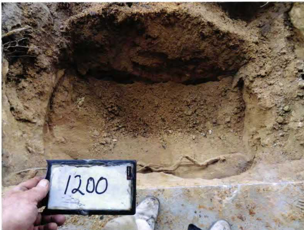
Picture 2: UST 1200Cardinal excavation.
